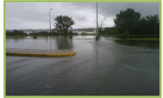
Figure 1. Post storm flooding in hospital parking lot.
